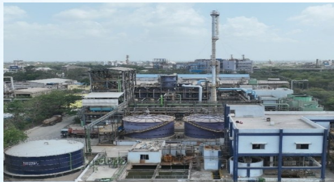
Sulphuric acid plant
