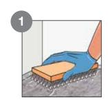
Ensure that the concrete surface is dry, clean and free of oil, grease and other contaminants. Remove any loose particles and dust using a wire brush.
