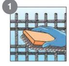
Ensure that the surface of the steel bars to be coated is dry, clean and free of oil, grease and other contaminants. Remove loose rust particles and dust using a wire brush.
