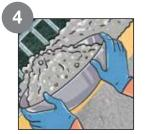
If the first coat is absorbed significantly, apply a second coat after 3 - 4 hour. Allow it to cure for 6 - 8 hour. While the Lapox® Lacrete coat is just tacky, apply the new concrete at this stage.
