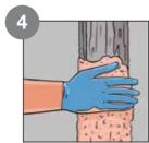
Press the mortar gently so that the crack is uniformly filled. For optimum results, allow it to cure for 48 - 72 hour.
