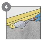
Thoroughly mix Lapox® Lacrete resin and hardener, in a 1:0.5 ratio, with 8 - 9 parts of Quartz Sand no. 10. Prepare the angle fillet (*watta*) 3 - 4 hour after applying the first coat.
