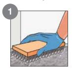
Ensure that the concrete surface is dry, clean and free of oil, grease and other contaminants. Remove any loose particles and dust using a wire brush.
