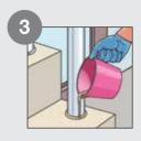
Pour the mixed material into the hole. It should be used within its pot life time.
