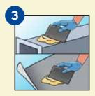
Apply Polygrip® HVAC adhesive range on both the substrates uniformly with the help of a brush or a spreader
